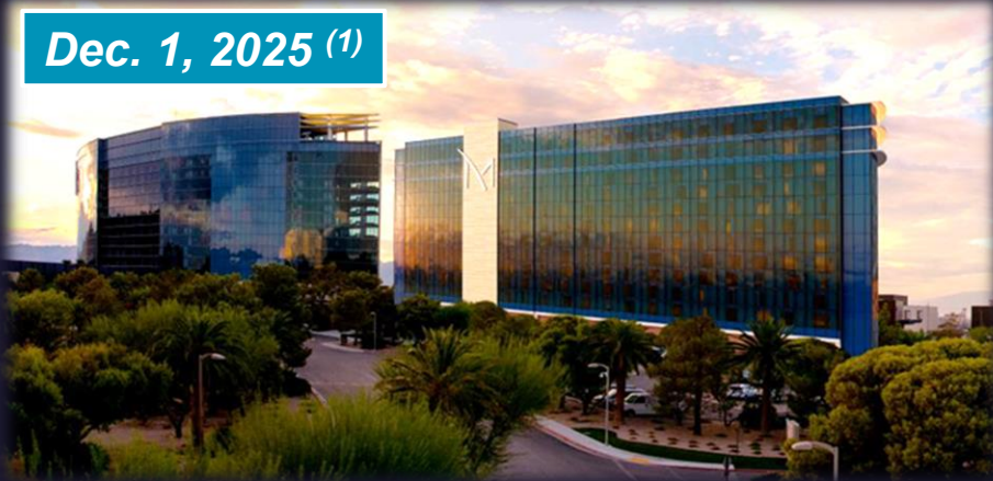
M Resort Hotel Tower
