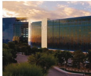
M RESORT ADDITIONAL HOTEL TOWER: 1H 2026
